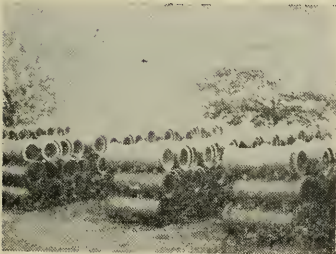
Sewer Line - Clay Pipe
