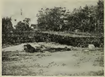
Cast Iron Pipes, Paper Mill Pond
