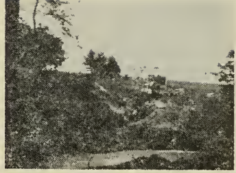
River Crossing, Collins St. 4 inch Water Main
