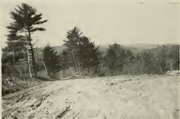
Town Dump After Grading
