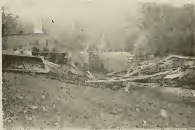
Debris Trapped by the Boom
