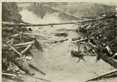
Debris in Channel
