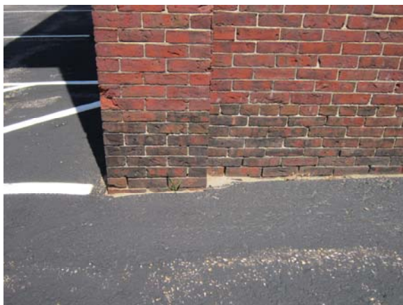
Figure 2 – Brick masonry at bottom of walls, especially those near pavement, exhibit substantial mortar loss due to roof water splashback.
