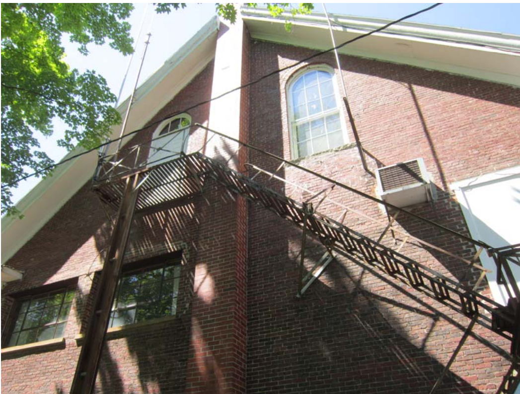
Previous renovations to the north façade include a fire escape with exit doors at the second and third floors, and steel windows punched through what was originally a blank wall.
