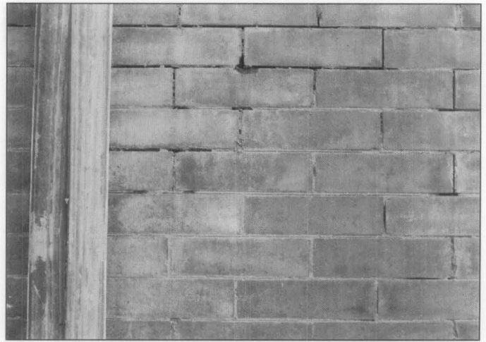
Figure 2. Much of the mortar on this building has been leached away by water from a leaking downspout. The downspout must be replaced and any other drainage problems repaired before repointing. Photo: Robert C. Mack, FAIA.
