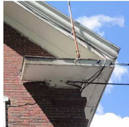
Figure 5 – Water and rodent damaged eave returns should be repaired or rebuilt.
