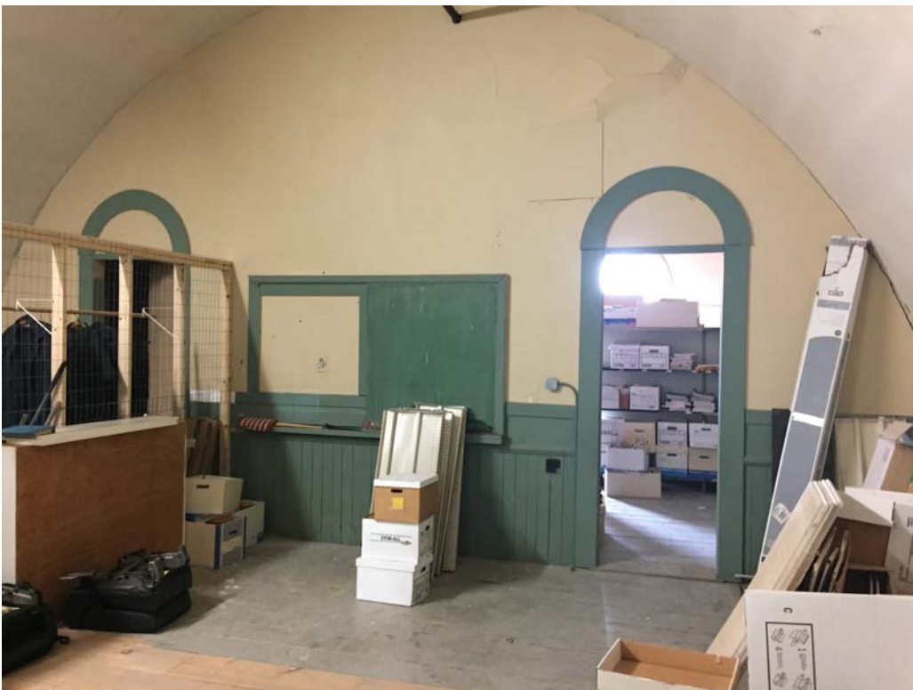
The entrance doors to the barrel-vaulted original second floor Hall (now the third floor and used for storage). The floor on this level will require reinforcement to support more than light storage.
