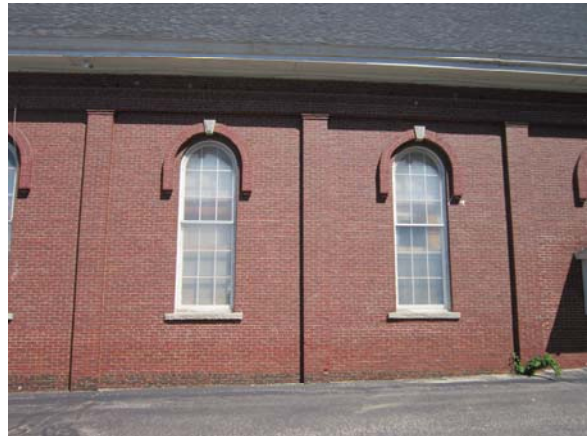
Figure 1 – Exposed foundation of slightly darker brick matches layout of wall brick above. Pavement on raised grade at south elevation conceals most of foundation.
