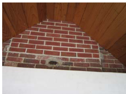
Figure 9 – Poor brick match at the inside of the existing north side portico.
