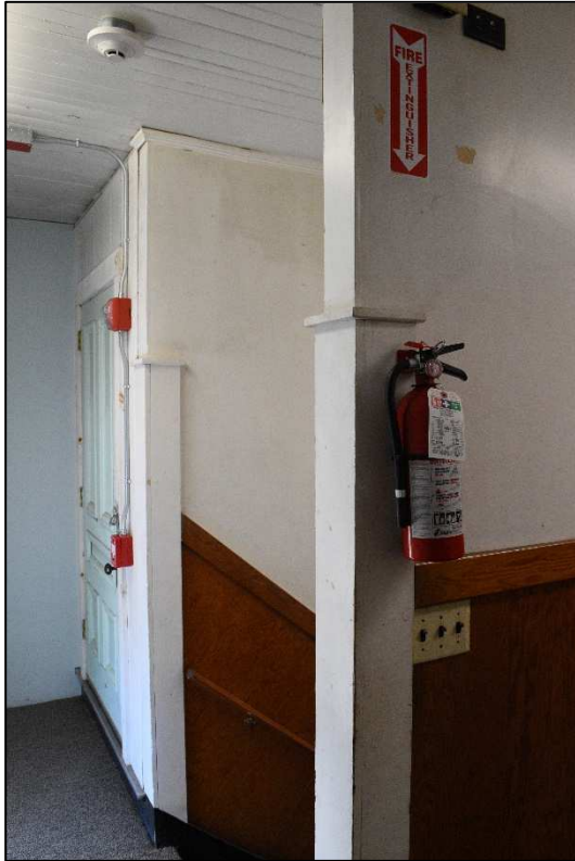
Figure 17: 1/2 newel posts at top of open stairway
