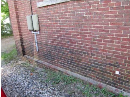
Figure 3 – Ten courses below the header course that marks the top of the foundation, Another header course caps a thickening of the foundation.
