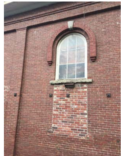
Figure 4 – Previous infill brick poorly matched to original brick – replace poor quality installation
