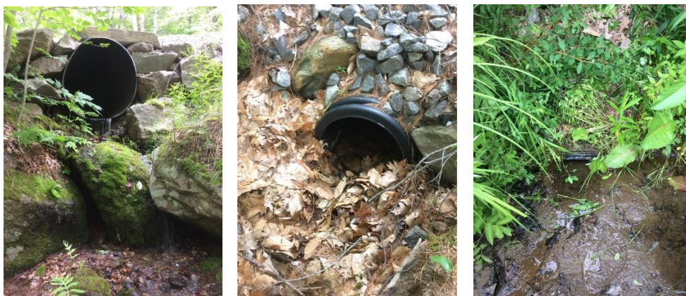
Figure 5: Examples of various amounts of sediment build up in Ashland, NH.
