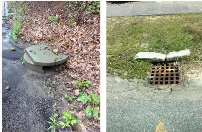
Figure 2: Examples of commonly found ‘Catch Basin Inlets’ in Ashland, NH. (Left: North Ashland Road near Route 3, Right: Highland Street near Cottage Street)
