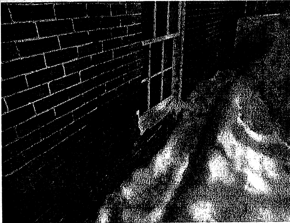
5-b damaged brick wall
