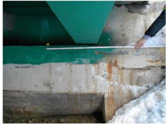
Abutment concrete spalling & cracking.
